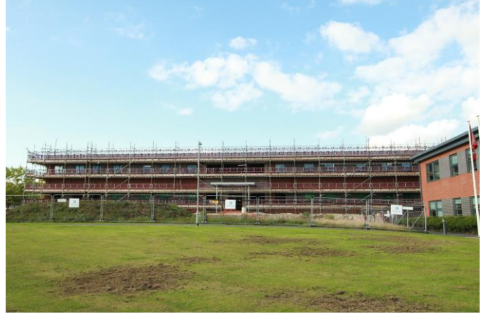
New RHQ construction
