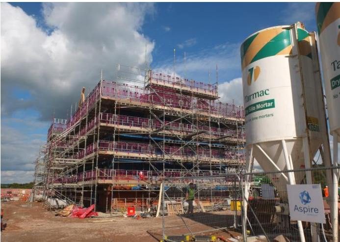
Construction of SLA at Bulford
