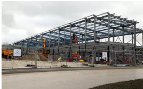
Technical Building, Purvis Lines
