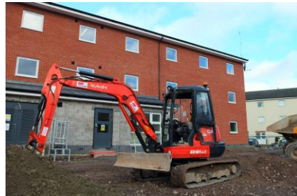
JRSLA construction at Tidworth
