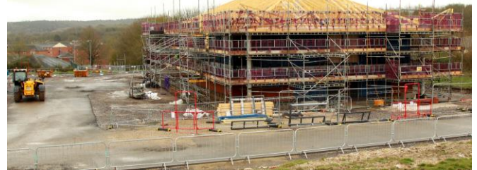
SNCO Mess - roof under construction
