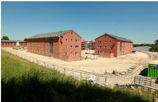
Single Living Accommodation under construction at Bulford during the heatwave
