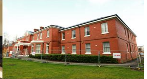
Refurbished Mess Tidworth
