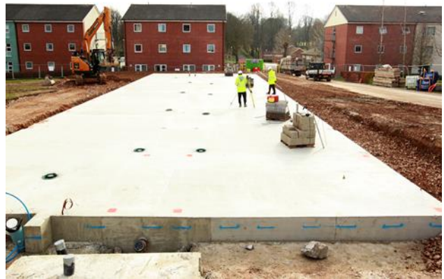
SLA Concrete Slab Preparation, Tidworth Feb 19
