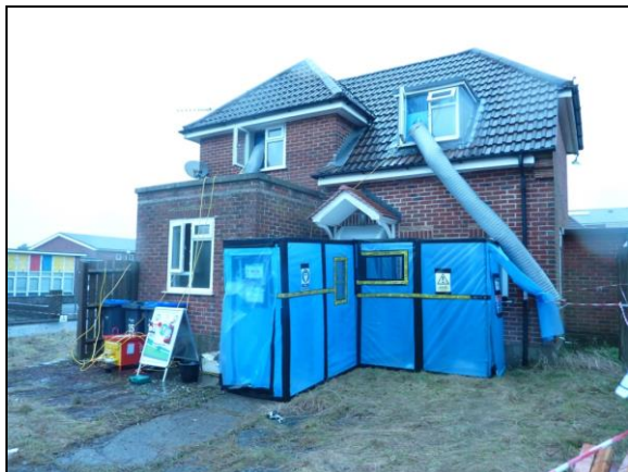
Asbestos removal from SFA
