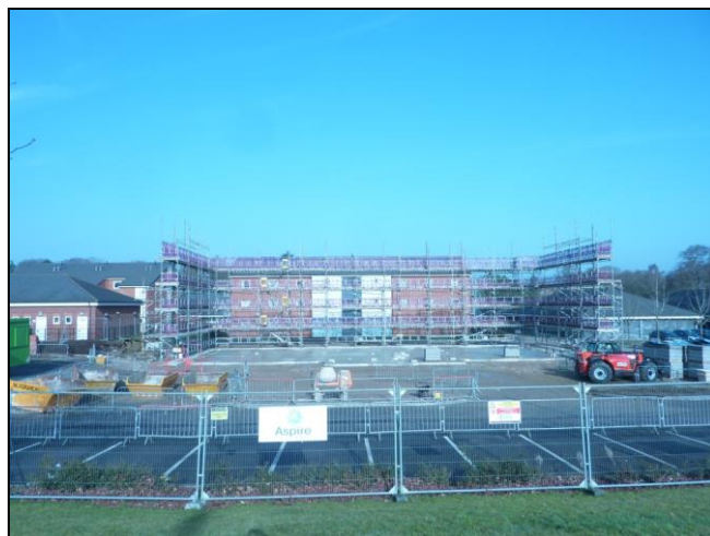
Preparation for SLA Modules at Aldershot
