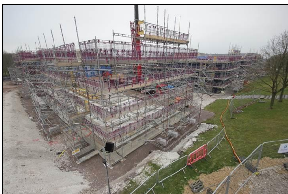
Progress on SLA at Larkhill
