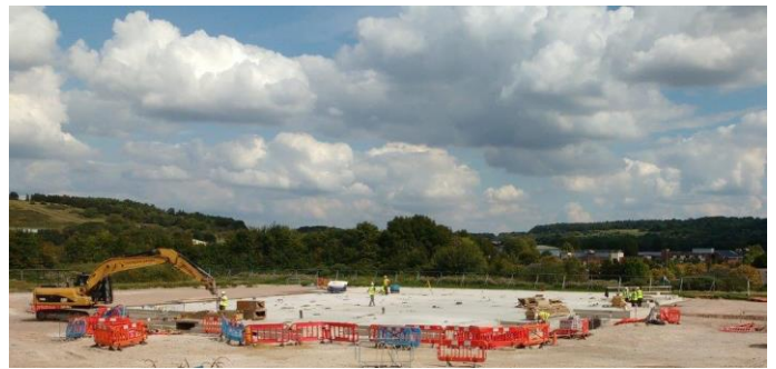
Completed slab at Tidworth
