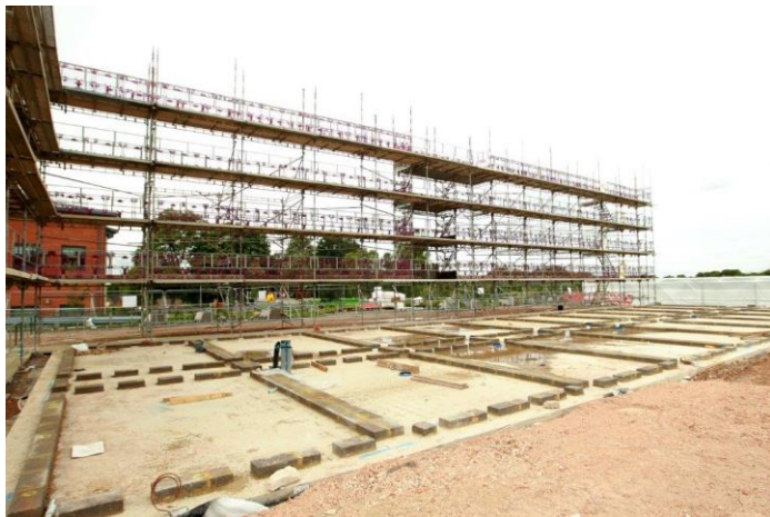
Construction of SLA at Bulford
