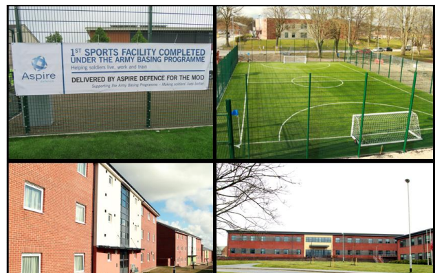
Delivery at Perham Down, clockwise from top left: 1 st sports facility banner; the new all-weather 5-a-side pitch; Junior Ranks' Single Living Accommodation; new Regimental Headquarters
