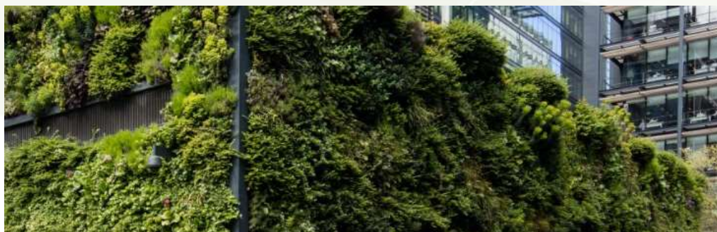
Image 3: Green walls, healthier cities, reduced run-off? (photo credit: UK Green Building Council)
