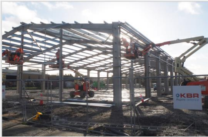
Technical Garage, Bulford
