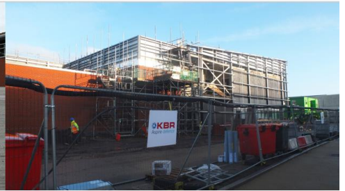
Physical Recreation Training Centre, Perham Down
